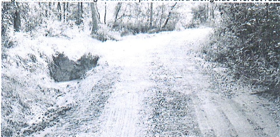
Figure 5K: A functioning sediment pit excavated alongside a forest road
