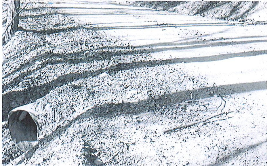
Figure 5H: View of the outlet end of a cross-drain installed underneath a permanent forest road in Wilkes County, N.C.
