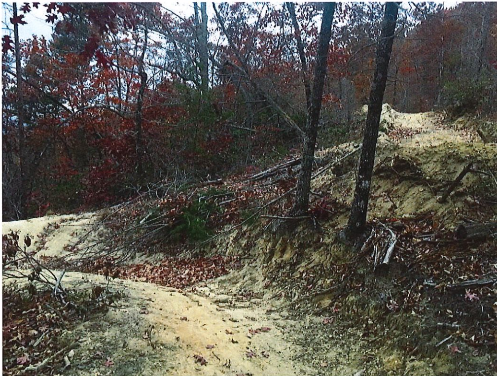
Figure 11. Dozer Line (center). Orphaned switchback (left).
