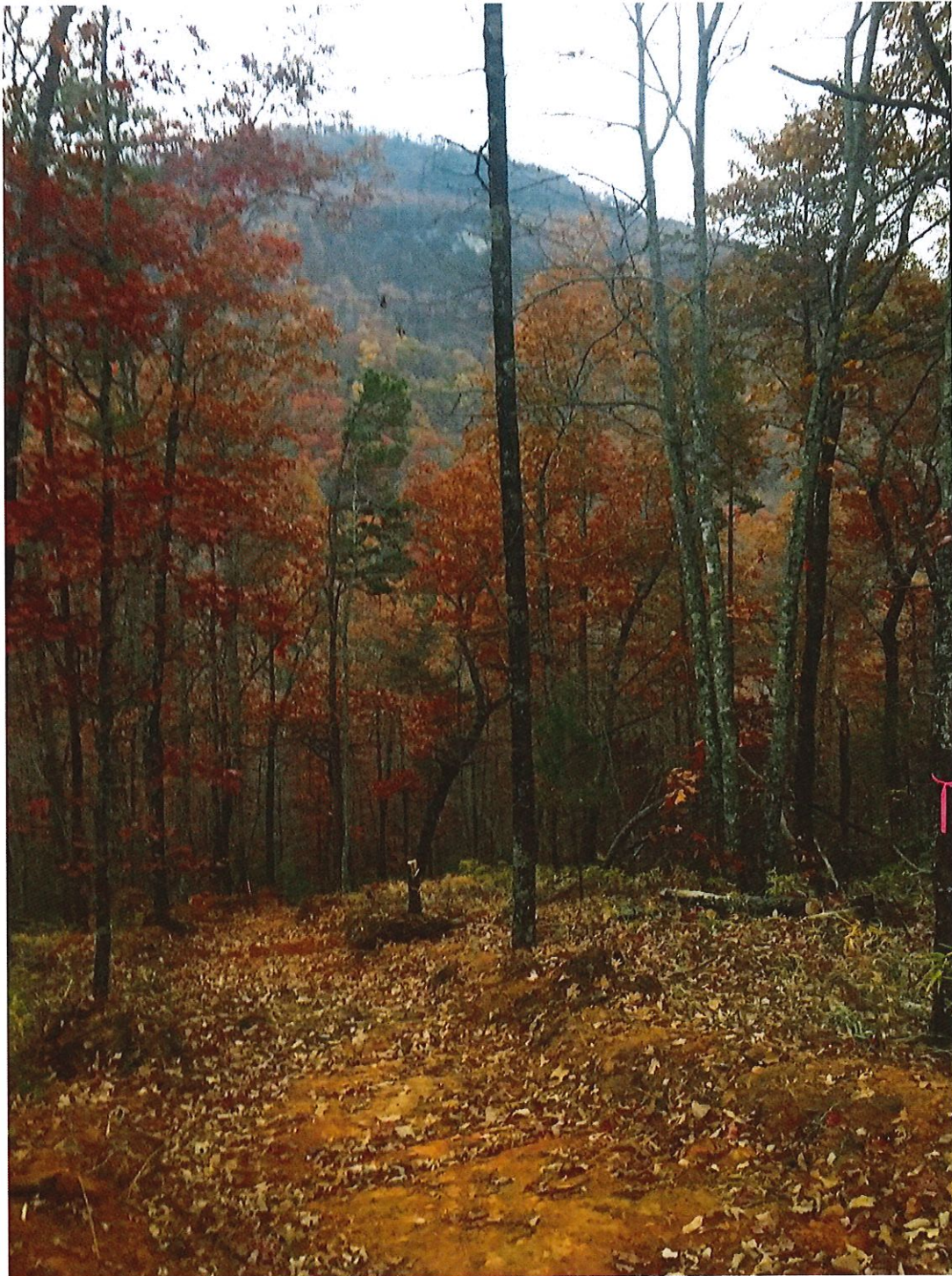
Figure 17. Dozer line significant below grade of natural ground will focus and accelerate water and sediment run-off. Wide corridor will entice trial users to follow open route.
