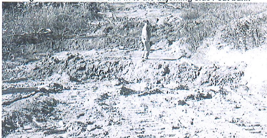
Figure 5D: A waterbar tied in to the adjoining side / cut bank
