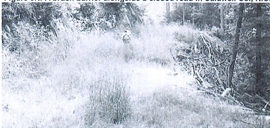
Figure 5O: A brush barrier at the base of an active road
