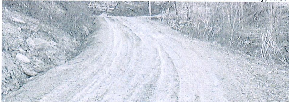
Figure 5G: A forest road with an inside ditchline in Ashe County, N.C.
