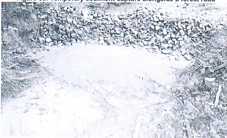
Figure 5J: Temporary sediment capture alongside a forest road
