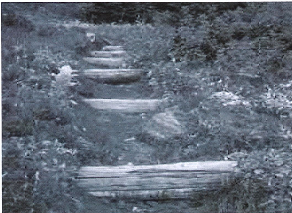
Figure 18. Example of wooden check dams; barriers can be constructed out of earth with machinery
