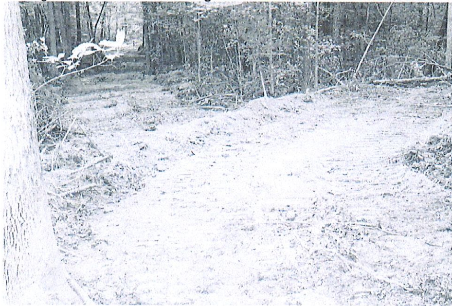
Figure 5E: A turnout used together with a waterbar on a skid trail
