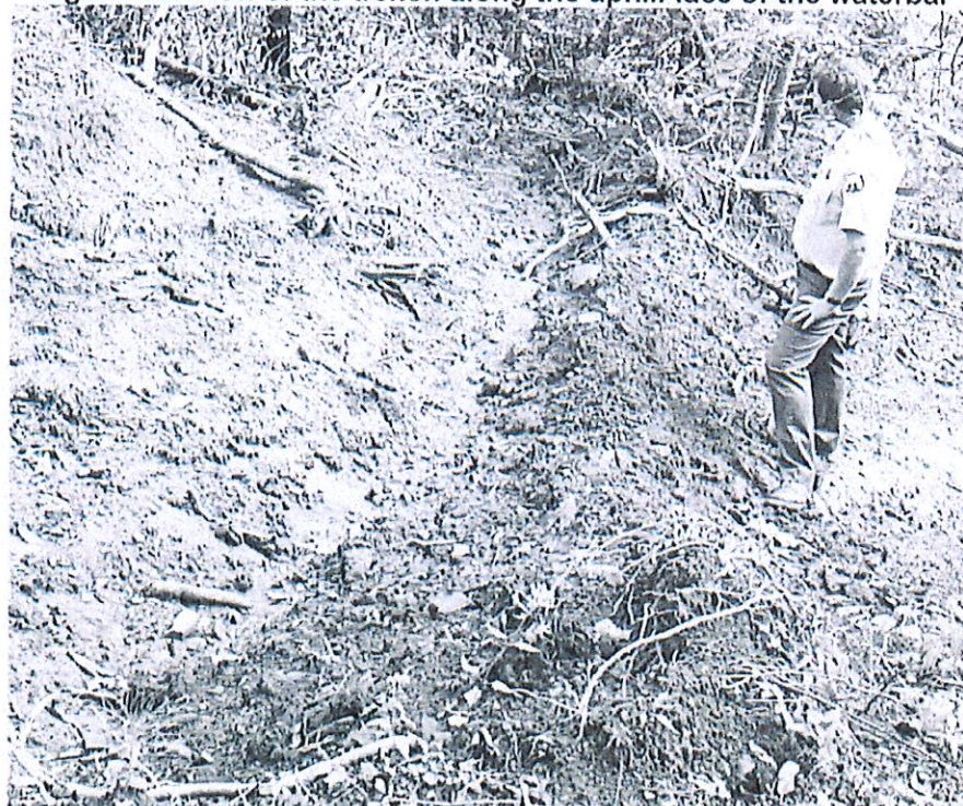
Figure 5C: View of the trench along the uphill face of the waterbar
