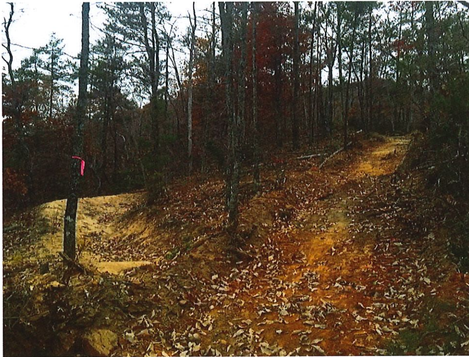
Figure 16. Dozer line (right center) at >30\% grade up fall line of ridge; Trail turn orphaned (left).
