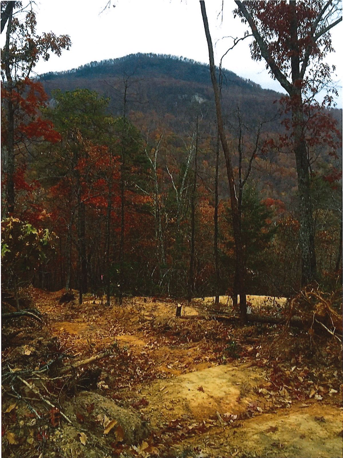
Figure 14. Steep dozer line has widened trail corridor considerably. Because 3-foot trail was perpendicular to dozer line, unvegetated corridor is up to 40 feet wide.
