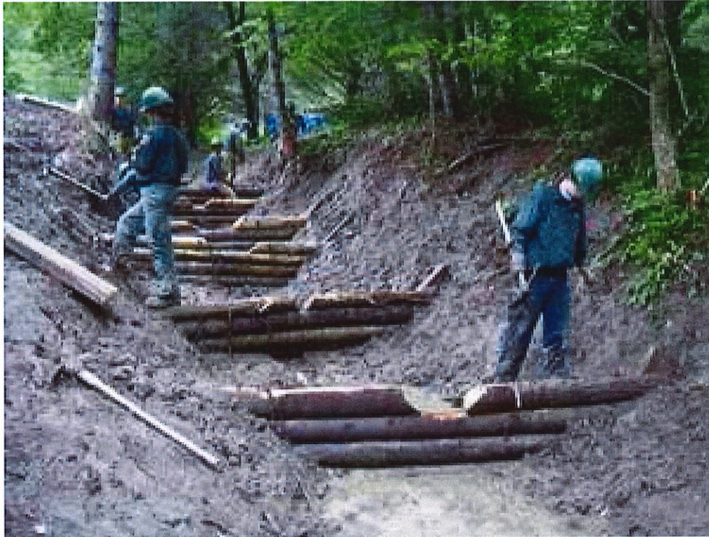
Figure 17. Example of wooden check dams; barriers can be constructed out of earth with machinery
