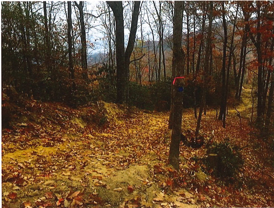
Figure 3. Upper section of trail widened to 8 feet, below grade for >500 feet of trail tread.
